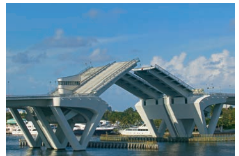
17th Street Causeway Bridge In Fort Lauderdale, FL. Exodermic® deck panels span floorbeams spaced at over 14 feet - composite with floorbeams and main girders.
