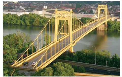
South 10th Street, sometimes referred to as the Philip Murray Bridge in Pittsburgh, PA was built in 1932 with a grid reinforced concrete deck that is still in service today!
