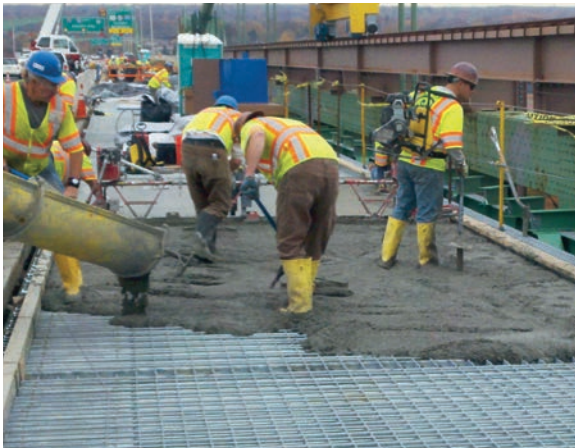
Walt Whitman Bridge deck installation in Philadelphia, PA Partial depth grid reinforced concrete deck replaced via CIP construction.
