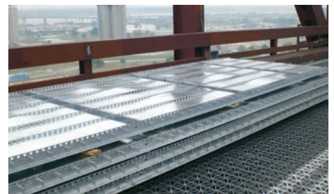
Grid deck panels for cast-in-place construction.
