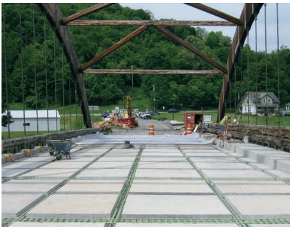
Robert C. Beach Memorial, or West Buckeye Bridge near Morgantown, WV. Precast Exodermic® deck panels prior to closure pour.
