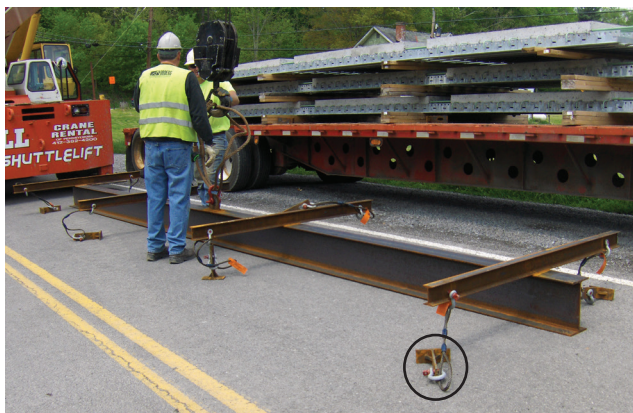
WT shape lifting device (circled).
