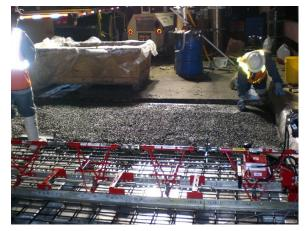
Mathews Bridge in Jacksonville, FL where lightweight concrete was used in conjunction with an Exodermic<sup>™</sup> deck to further reduce weight. The deck weighs less than 50 pounds per square foot while maintaining 2 inches of concrete cover over the rebar.
